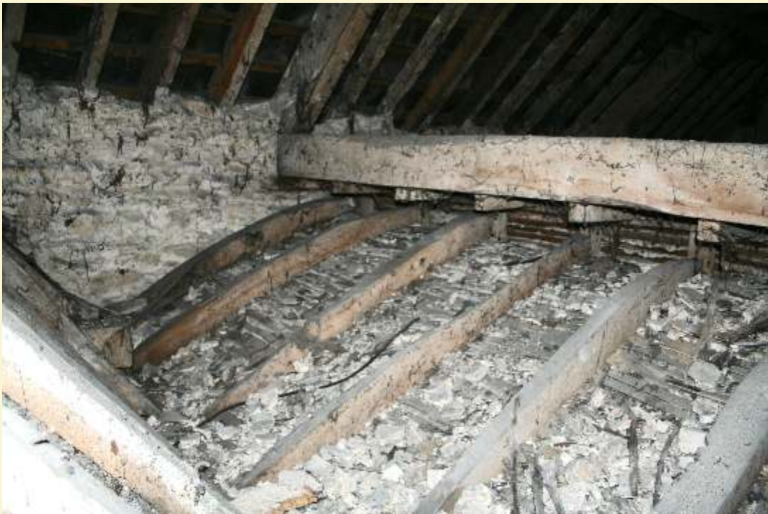
A coved ceiling to one of the upper floor rooms is typical of Georgian improvements. This is the supporting structure viewed from the attic.
