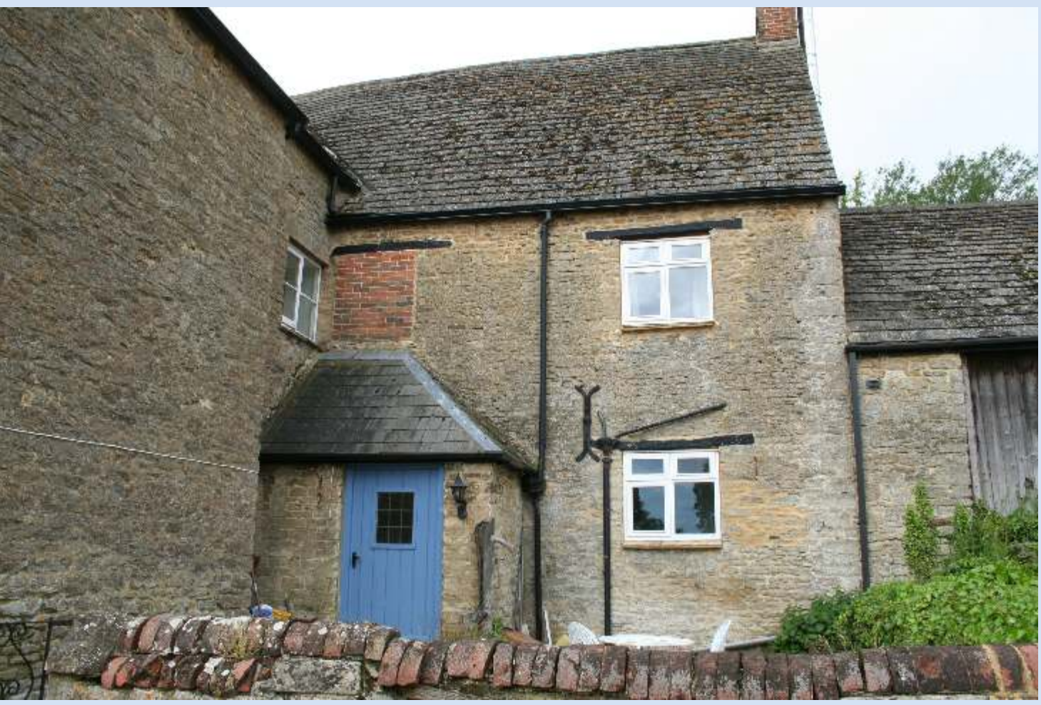
The re-entrant showing how Bay B masters the rear wing; note also the blocked first floor window.
