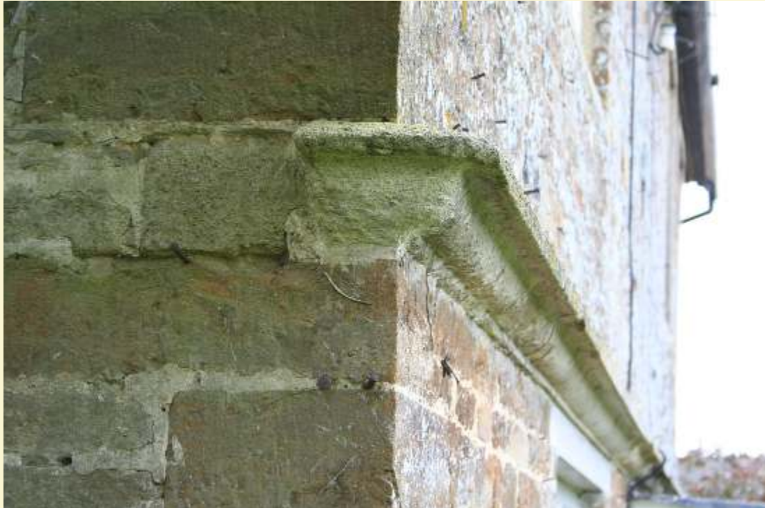
The string course on the frontage returns on the right gable end, but not on the left one.
