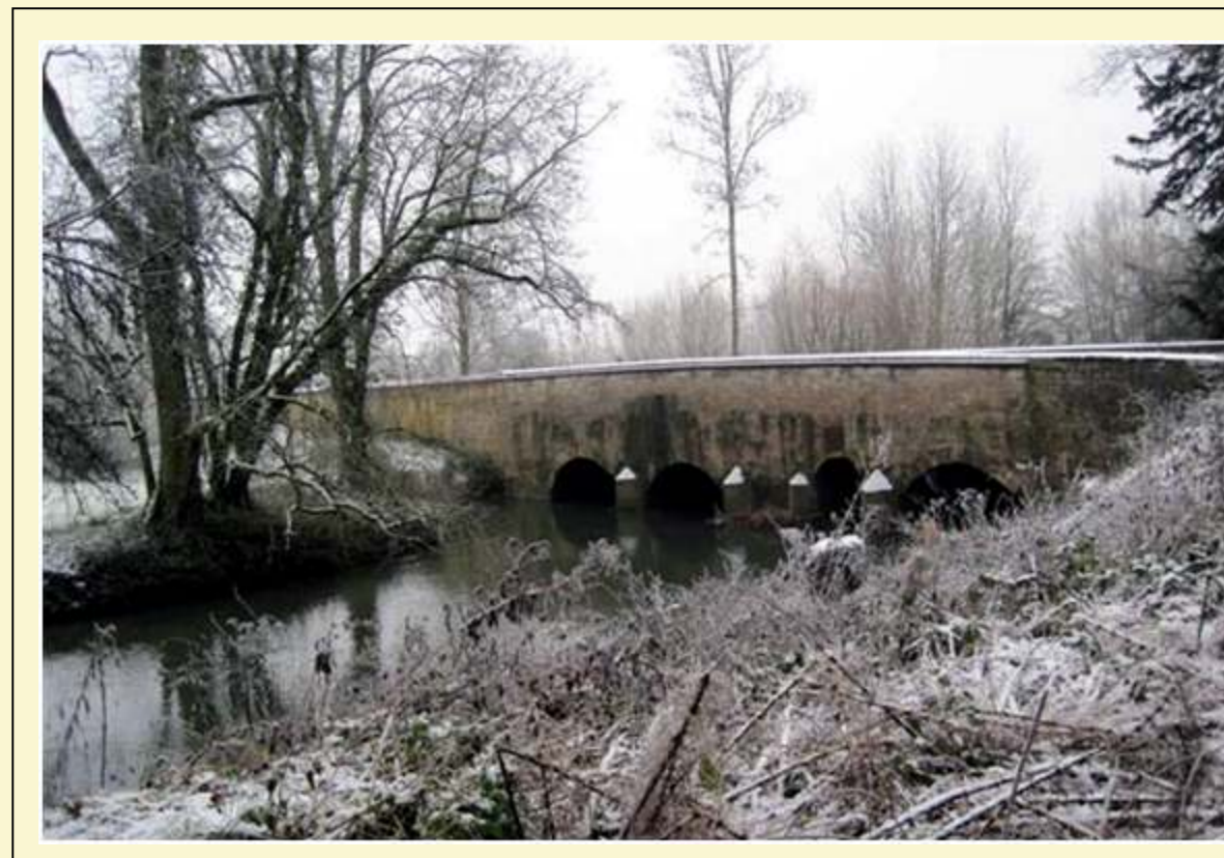
SAL – Apr 1995 BRIDGE REPAIRS
